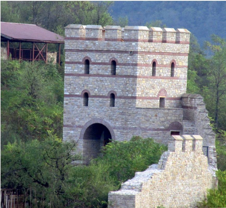
FIGURE 14 The northern tower of Trapezitsa. AUTHOR'S PHOTO.
